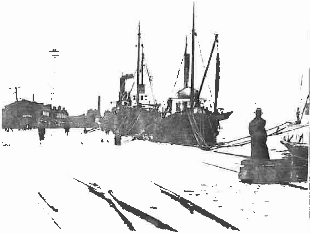
a) Wharf Being Overtopped, Mawhera Quay, Looking Downstream. (W.C.B.).
